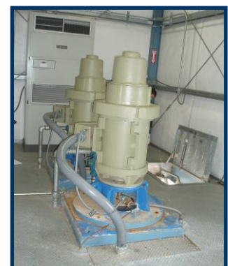
Photo 3: South River Pump Station
