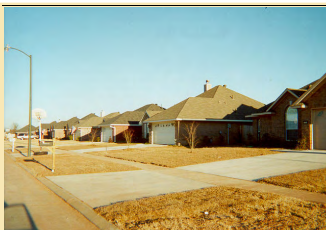
New developments inside the City have curb and gutter streets, sidewalks, and streetlights.
